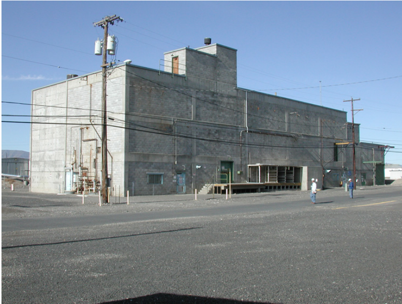
224-B Plutonium Separation Plant, Hanford, WA, 1985
