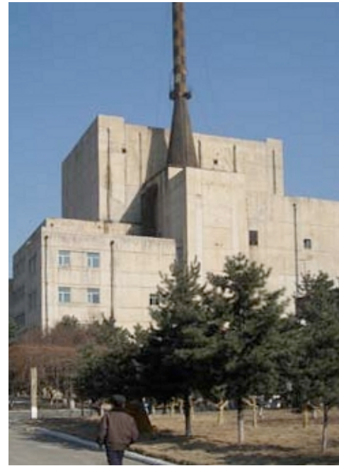
Reactor, Yongbyon, NK
