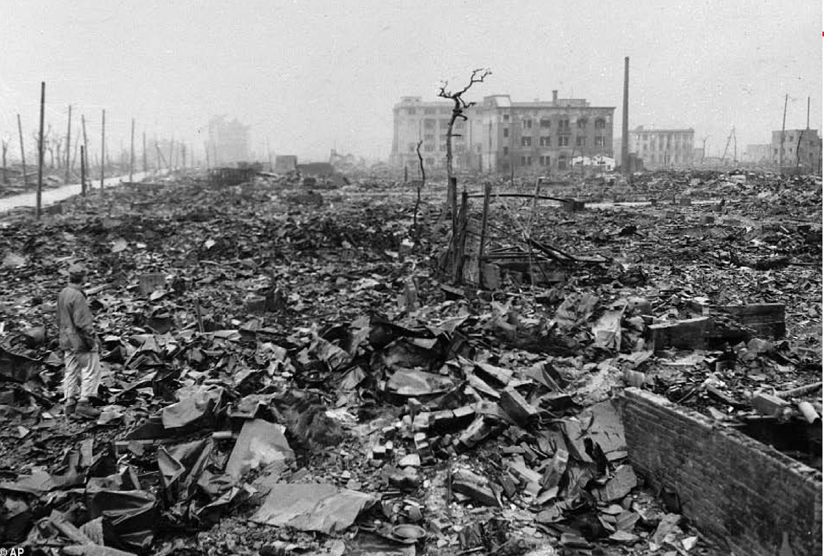
Impact of the 15 kiloton detonation in Hiroshima on wood-framed structures
