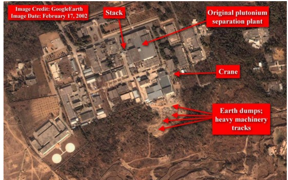
Plutonium Separation Plant Rawalpindi, Pakistan, Feb 2002
