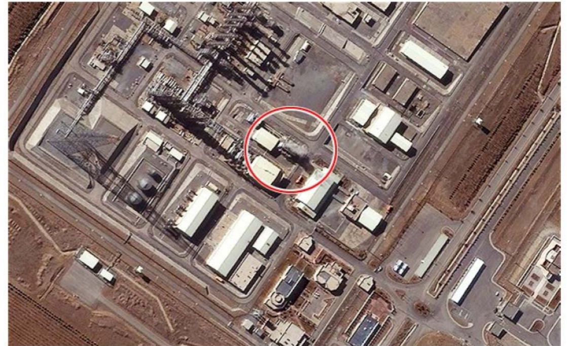
Water vapour, circled, is seen being emitted from forced air coolers at the Arak heavy water production plant earlier this month, showing that the facility is operational Photo: DigitalGlobe Inc/McKenzie Intelligence Ltd
