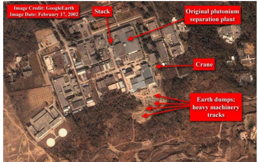
Plutonium Separation Plant Rawalpindi, Pakistan, Feb 2002
