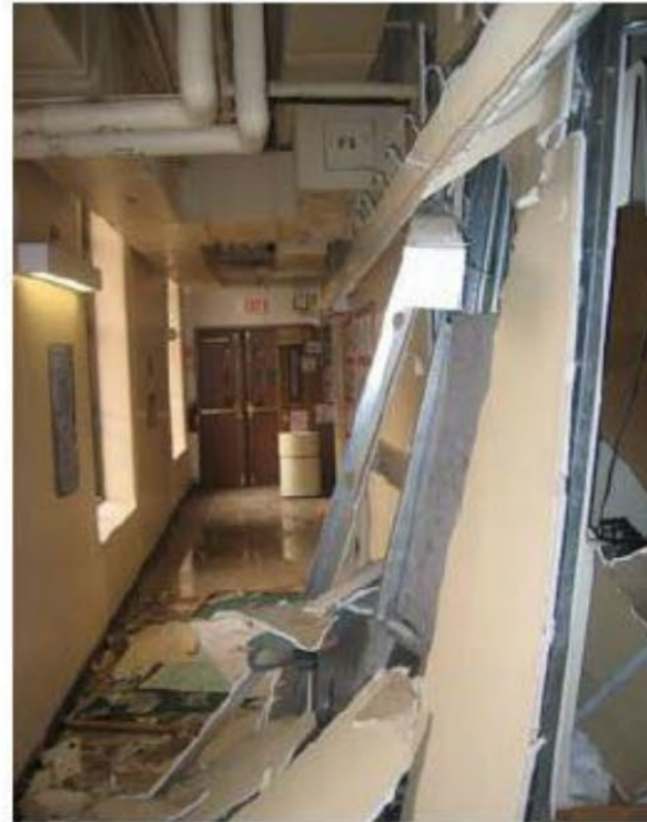
Figure 2 - Hallway Outside Laboratory Showing Explosion Damage
