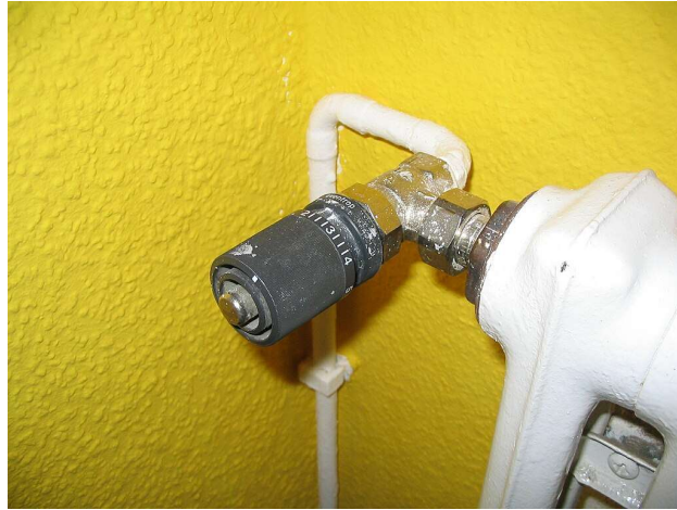
Fig. 1.5: Example of heating radiator thermostatic control valve.
