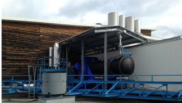
TS Condenser: 15m above ground level (92m above ATLAS): Condenses 1.2 kg/s C_3F_8 using cold liquid C_6F_{14} Pumped up at -65\text{ }^\circ\text{C}
