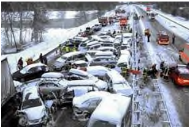
Cascading failure on "high-performance" road
