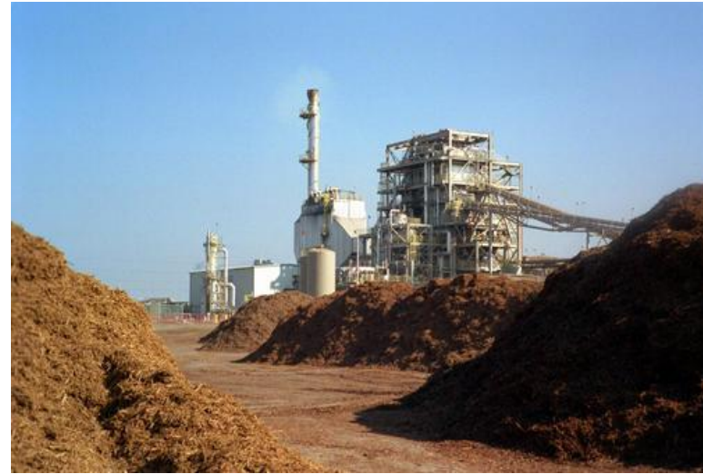
21 MW Tracy Biomass Plant
