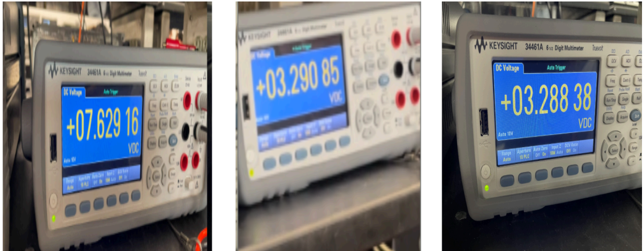
Figure 3. Power Subsystem Voltage Measurements (Battery Power Supplied, Voltage Regulator Output, Voltage Regulator Output During Siren Activation)
