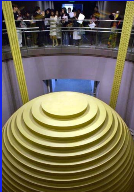
Tuned mass damper (pendulum) in Taipei 101
