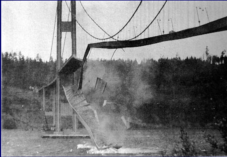
Tacoma Narrows Bridge
