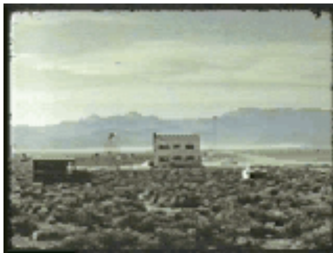
Effect of a 16 kt explosion on a house 1 mi away (equivalent to a 1 Mt explosion on a house 5 mi away, but happens 10x faster)
