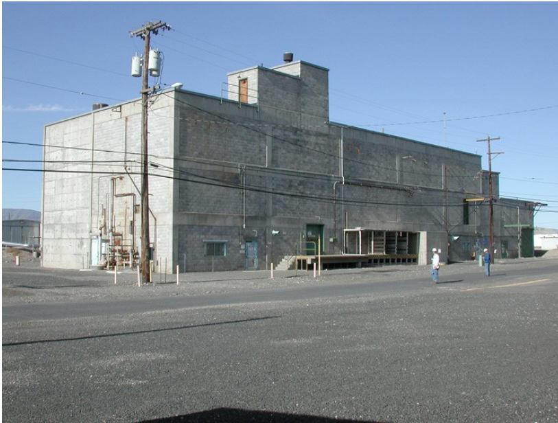
224-B Plutonium Separation Plant, Hanford, WA, 1985
