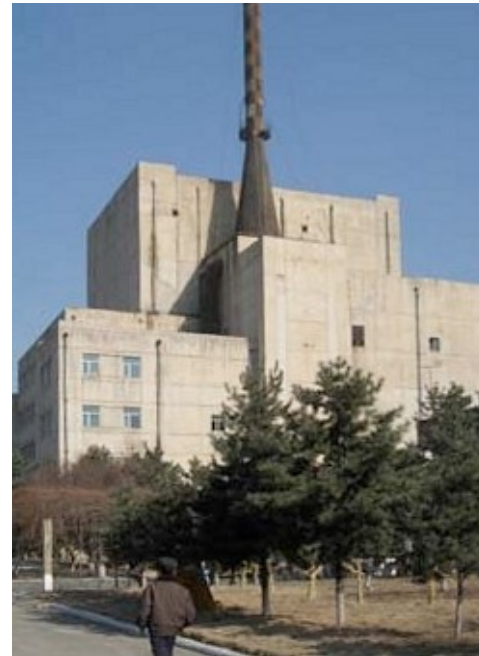
Reactor, Yongbyon, NK
