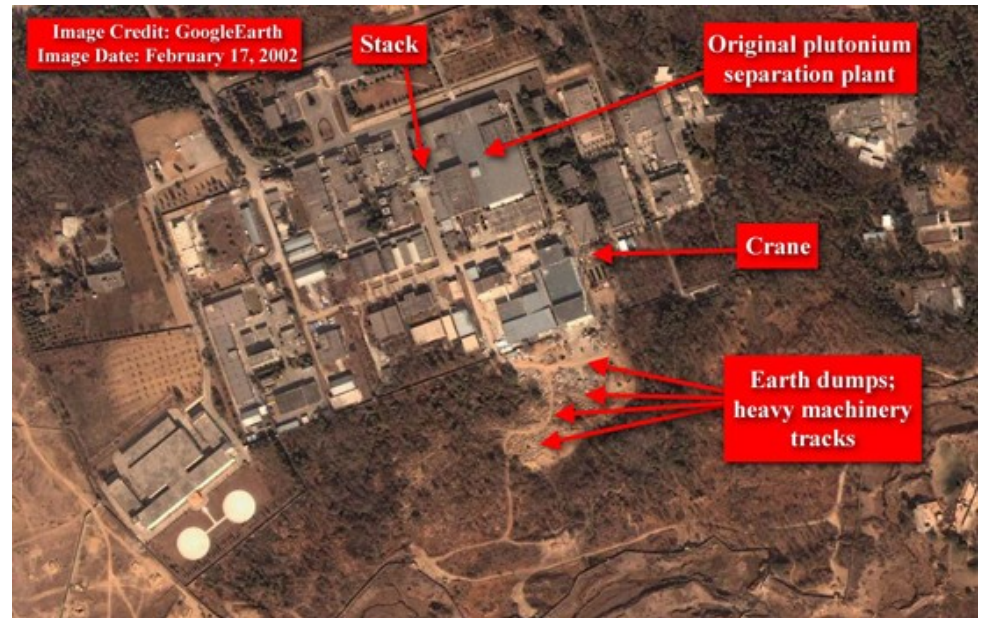
Plutonium Separation Plant Rawalpindi, Pakistan, Feb 2002
