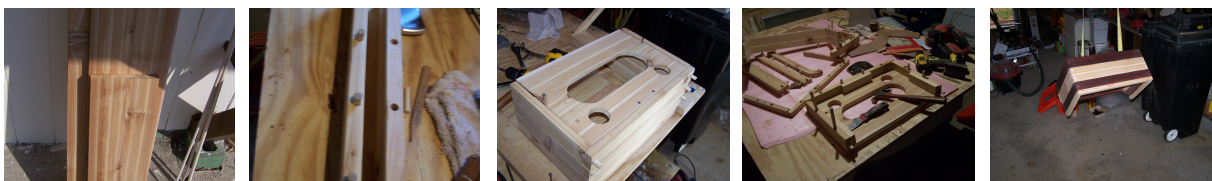
Images from the enclosure building process
