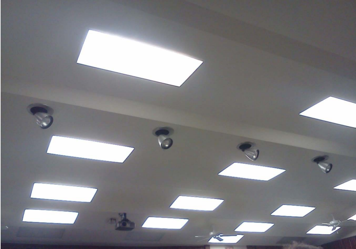
Figure 6 The ceiling has a saw-tooth profile, angled to reflect towards the speaker
