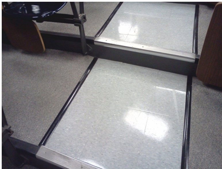
Figure 5 The floor is carpeted with exception to the tile paths
