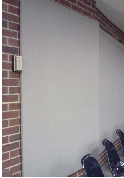
Figure 7 Acoustical panel along back walls for sound absorption
