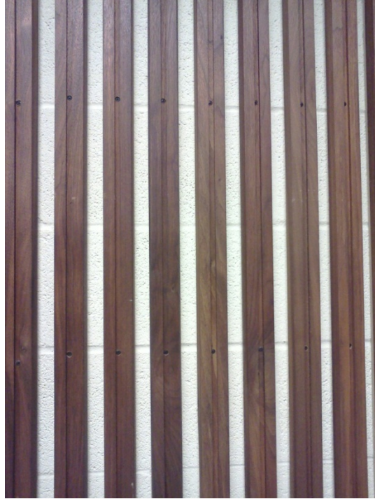
Figure 4 The wooden boards attached vertically to the walls to entrap and/or diffuse sound
