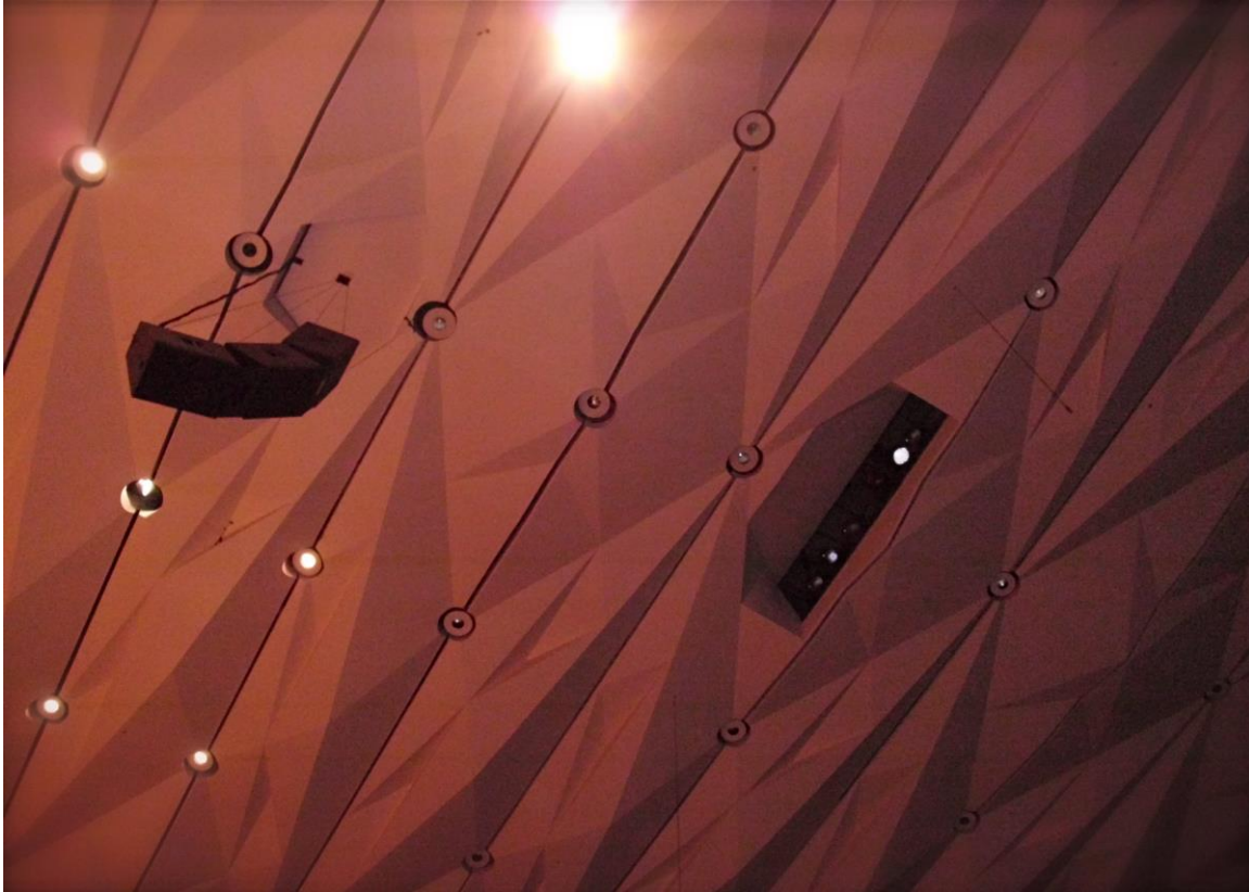
Figure 3: Tiered Ceiling (Plaster Suspended From Springs).
