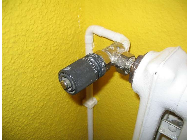
Fig. 1.5: Example of heating radiator thermostatic control valve.
