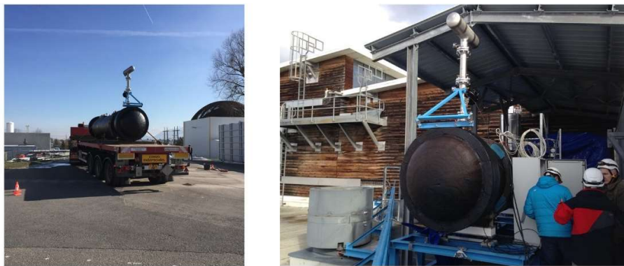
Fig 3.8: Installation of the condenser of the ATLAS thermosiphon on the roof of the CERN LHC Point 1 facilities building (15 meters above ground level, 92 meters above the ATLAS experimental cavern).
