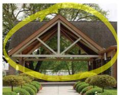
Trusses are commonly used to support roofs.
