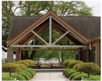
Trusses are commonly used to support roofs.
