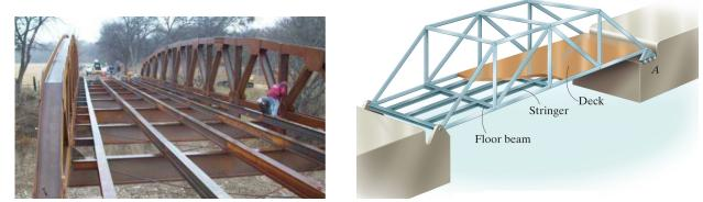
To analyze the design of a truss, we will work through a **free-body diagram** including **reaction forces**, followed by **equations for equilibrium**, and determine **reaction forces at the sup-ports** and **internal forces** on the supporting side truss members. For everything ahead, we will simplify the problem by considering it in 2D.
